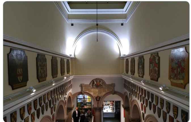
LED lighting in the main hall
